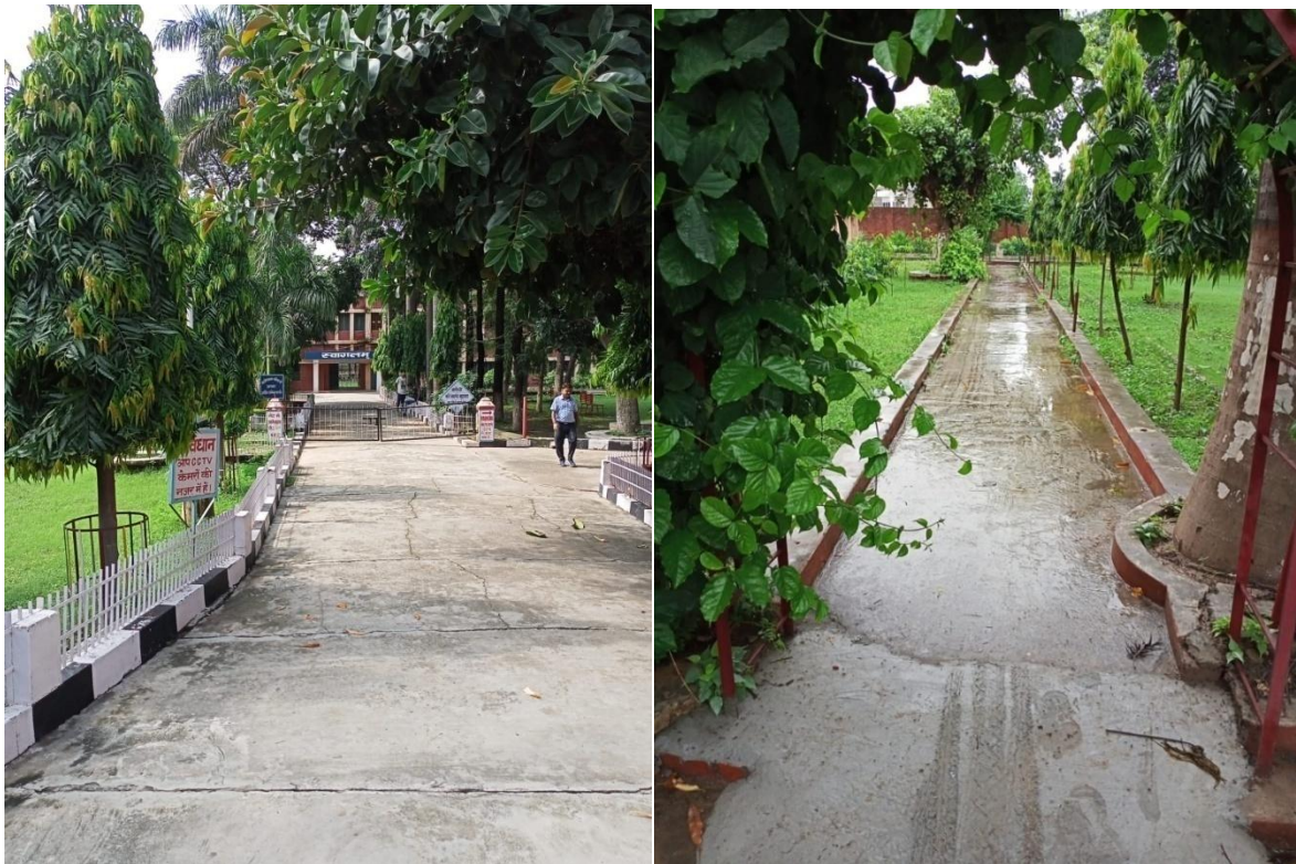
Concrete Pedestrian Pathway
